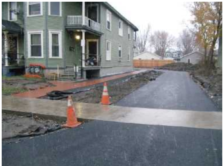
New Porous Paver Walkway and Driveway to Porous Parking Area
