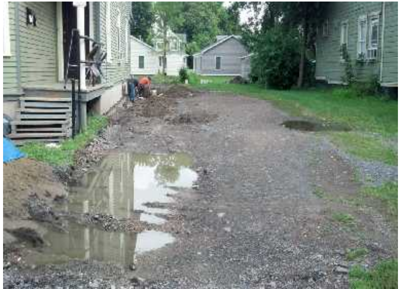
Site Conditions Prior to Construction
