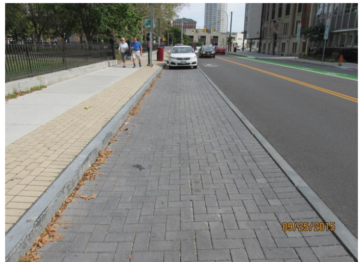
Porous Paver Parking Lane and Snow Storage Area on East Genesee Street at Forman Park
