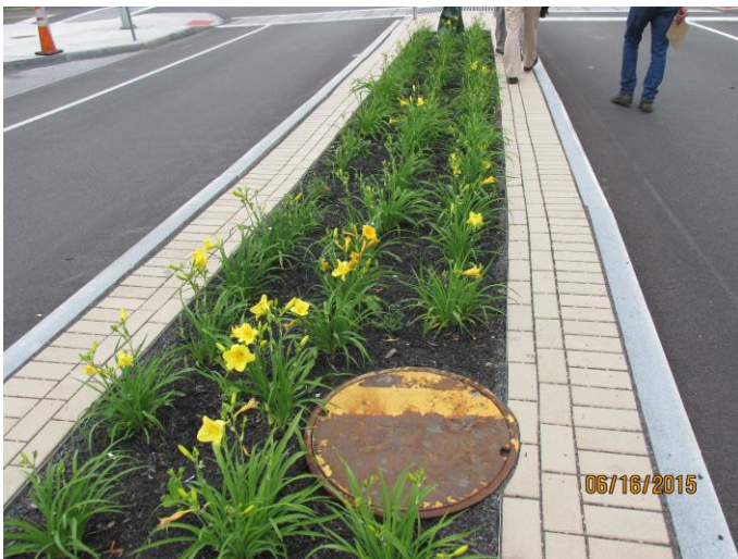
Porous Pavers and Plantings within East Genesee Street Median
