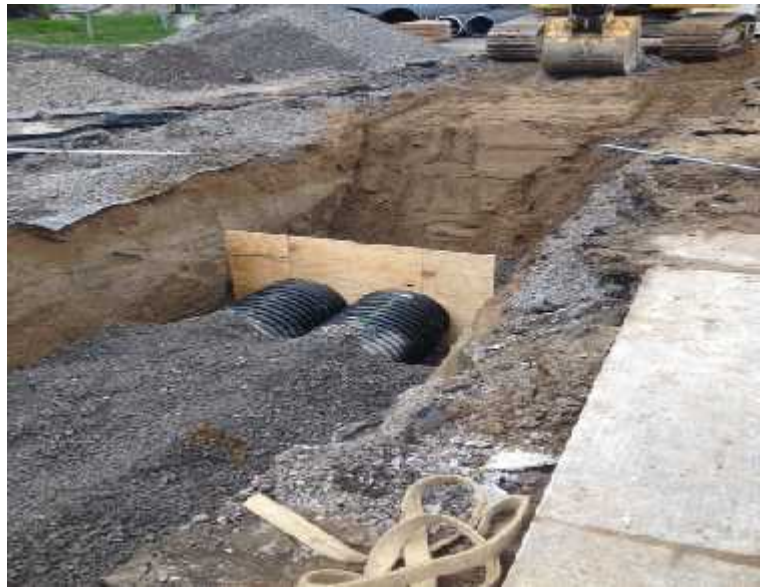
Installation of the Subsurface Infiltration Trench
