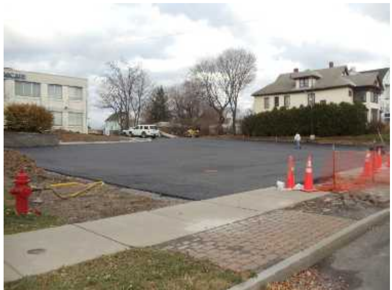
New Drive Lane with Sub-Surface Storage Chambers
