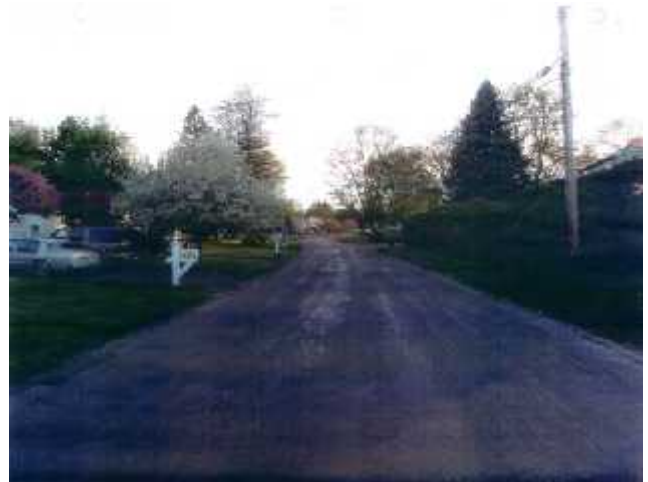
Project Site BEFORE Construction
