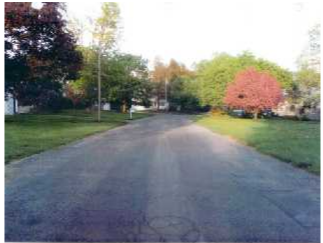
Project Site BEFORE Construction
