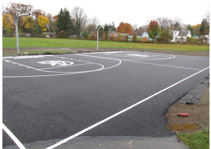
Completed Porous Asphalt Basketball Court
