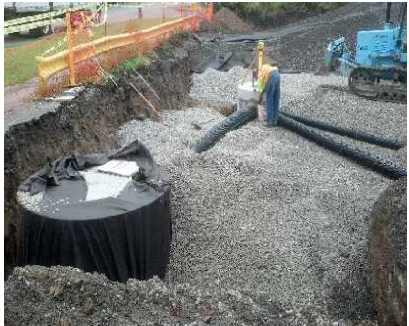
Construction of Subsurface Infiltration System
