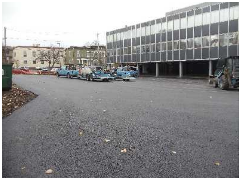
New Parking Area Above Subsurface Infiltration System
