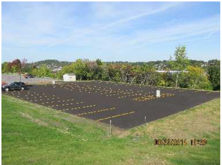
Parking Area Featuring Porous Pavement Parking Lanes
