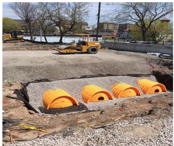
Installation of Underground Infiltration System
