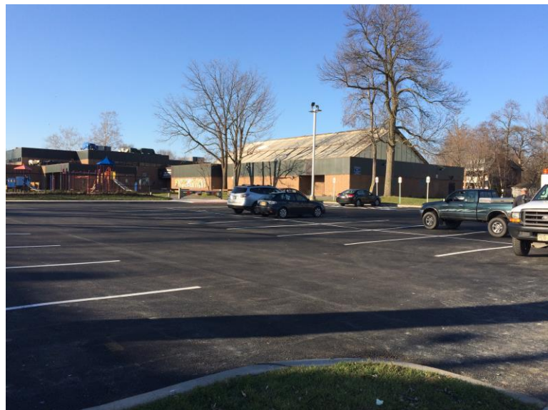
Improved SWCC parking lot with porous pavement for stormwater infiltration
