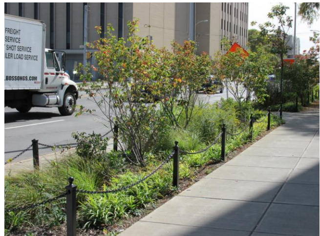
Example Rain Garden, State Street
