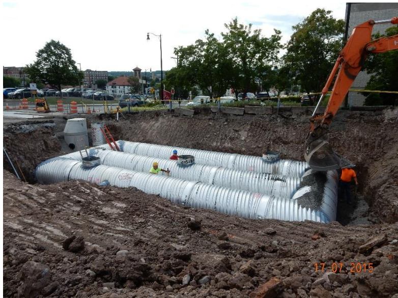
Installation of Underground Cistern/Chamber System
