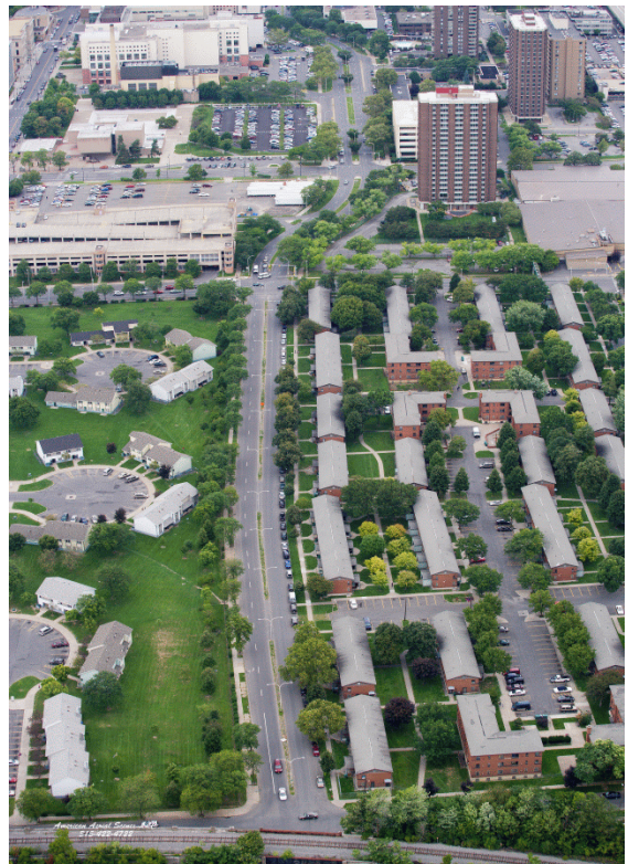
Aerial View of Townsend Median after Retrofit (Facing North)
