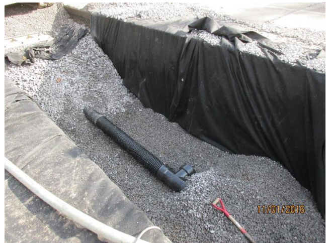
Underground Infiltration Trench installed on Lynch Avenue
