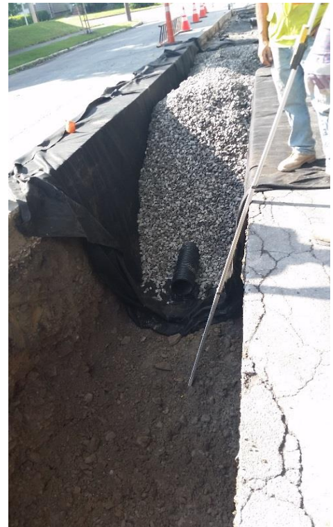
Construction of an Infiltration Trench on Wellesley Road (August 2017)
