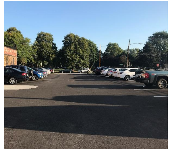
Parking Lot Above Underground Detention Basin
