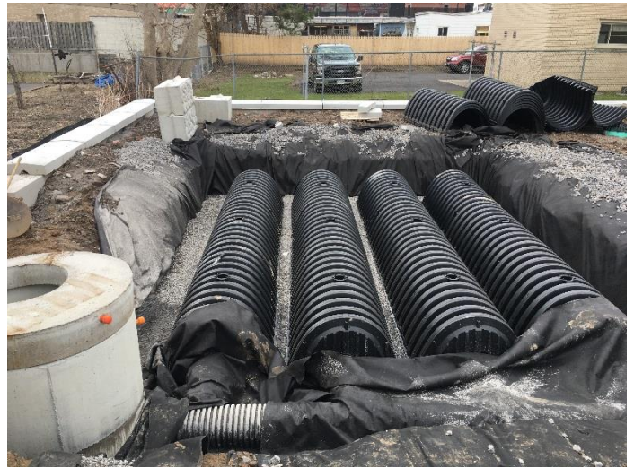
Construction of the Underground Infiltration
