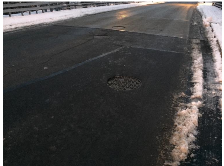
Photo of the Project Area after Construction at Newell Street, Looking West
