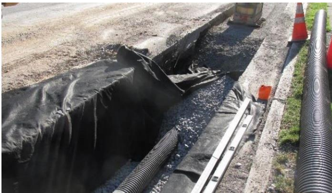
Typical Underground Infiltration Trench
