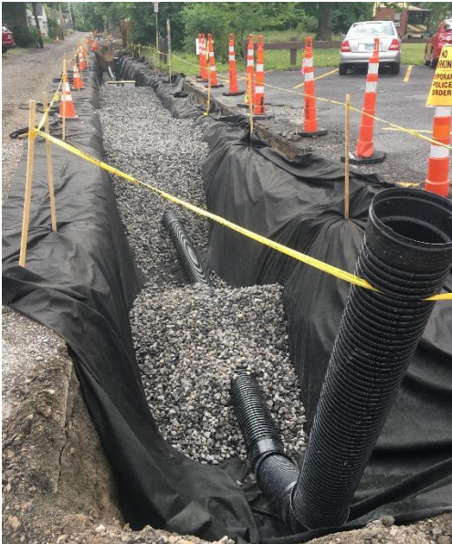
Construction of the Infiltration Trench (July 2018)
