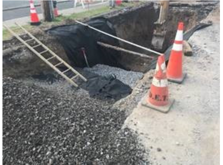
Underground infiltration trench installation on South Avenue
