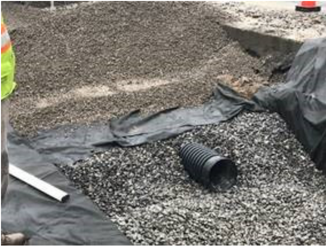
Underground infiltration trench installation on South Avenue
