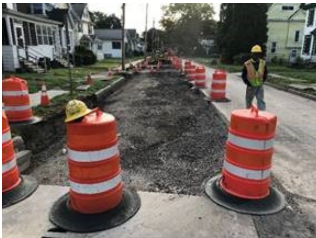
Completed infiltration trench awaiting new pavement on Elmhurst Avenue
