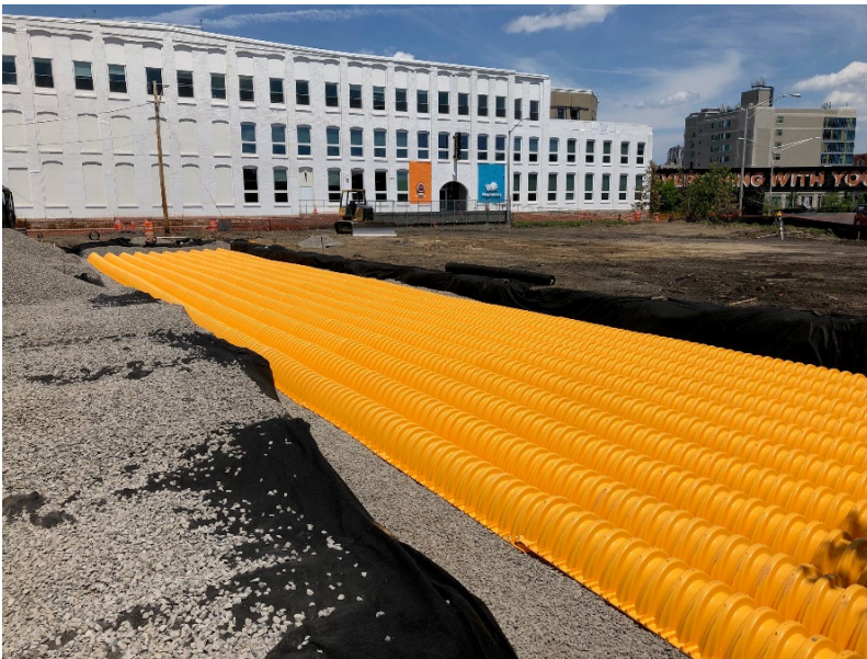
Construction of the underground storage chamber infiltration trench system
