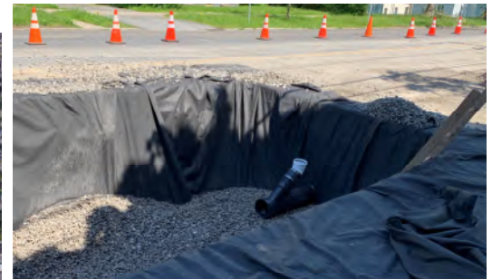
Wilbur Avenue Infiltration Trench
