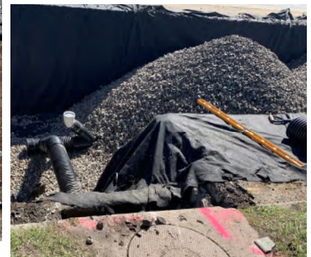
Wilbur Avenue Catch Basin to Infiltration Trench
