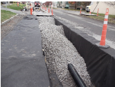
Example Underground Infiltration Trench
