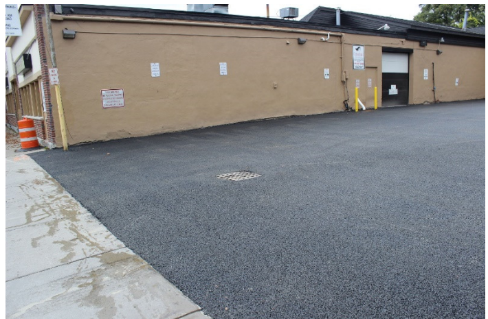
Completed porous pavement parking lot
