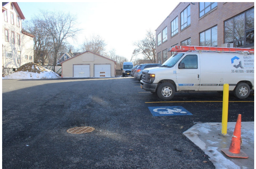
New porous asphalt parking lot at North Side Learning Center
