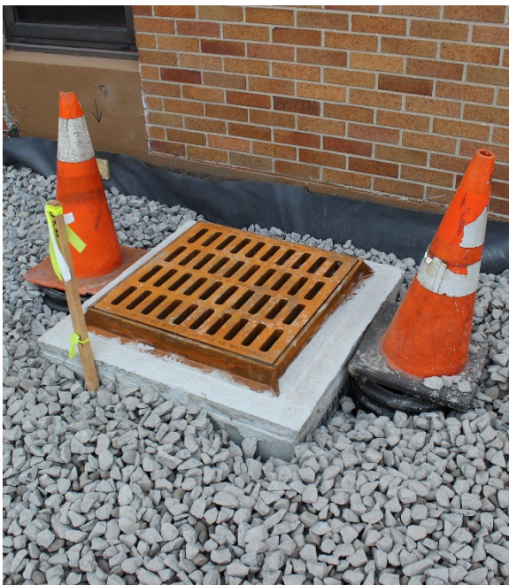
Newly installed catch basin in parking lot
