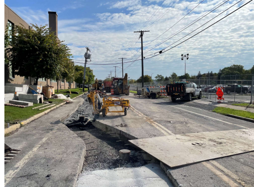
Construction of the East Water Street Road Reconstruction Green Infrastructure Project
