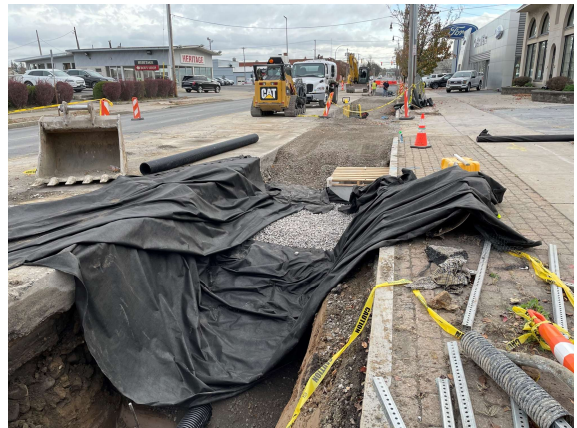
Construction of an Infiltration Trench on West Genesee Street in CSO 066
