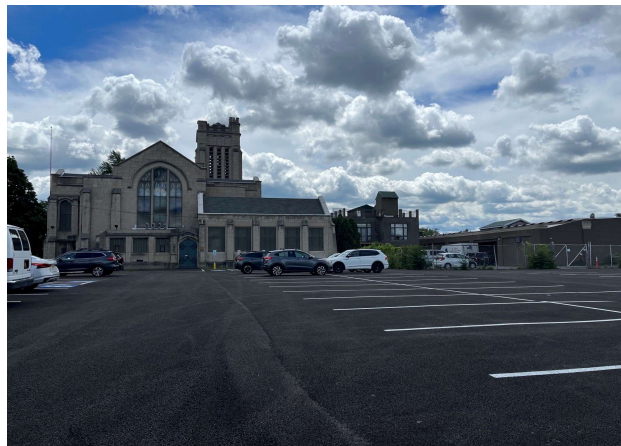
Construction of the Missio Church GIF project in CSO 066 was completed in 2022 and featured a porous asphalt parking lot and added green space
