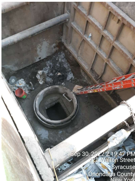
Construction of the CSO 029 Abatement Project (left) and photo of the new CSO 029 Regulator Structure (right)
