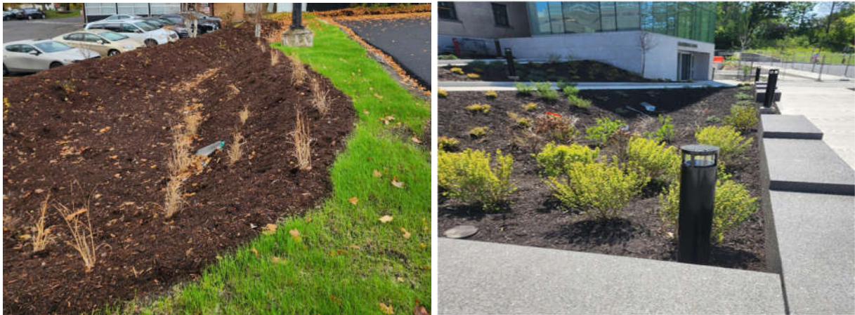
Photographs of the Interfaith Works GIF project’s porous pavement parking lot and bioretention (left), and the ESF GIF project’s bioretention areas (right).
