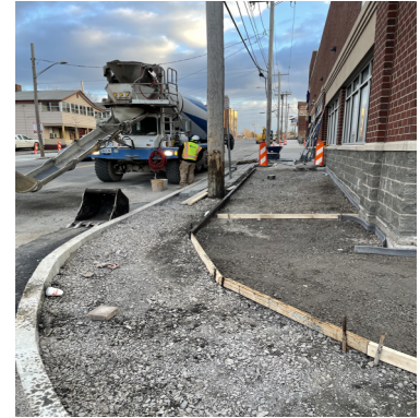
Construction of the Butternut Street Green Corridor Project
