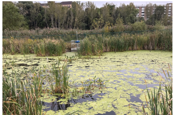
Harbor Brook CSO 018 Constructed Wetlands Storage and Treatment Facility
