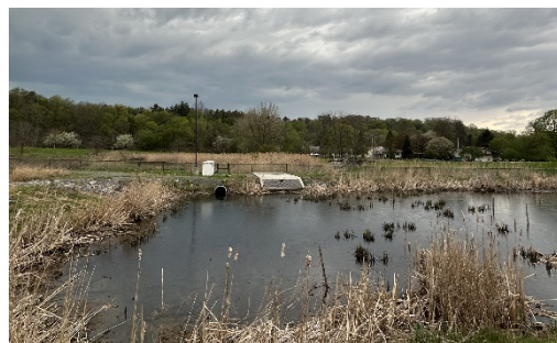
Harbor Brook CSO 018 Constructed Wetlands Storage and Treatment Facility
