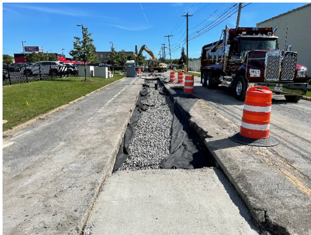
Construction photos of the underground infiltration trenches on East Water Street
