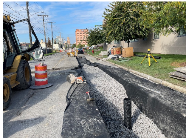
Construction photos of the underground infiltration trenches on East Water Street
