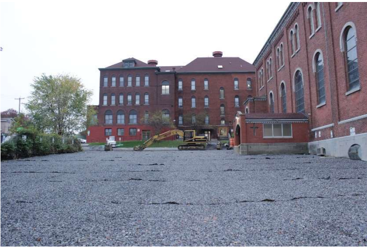
View of the porous lot under construction at the Assumption Church
