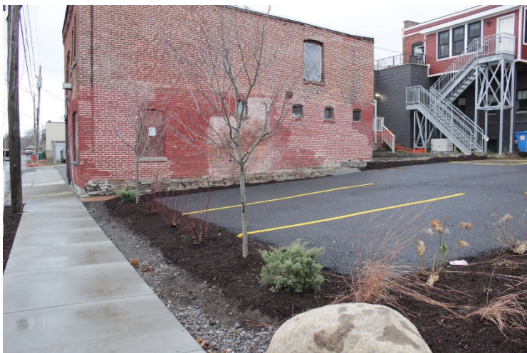
Partial view of the 701 N Salina St Project. The porous parking lot is generally surrounded by added green space and porous pavers
