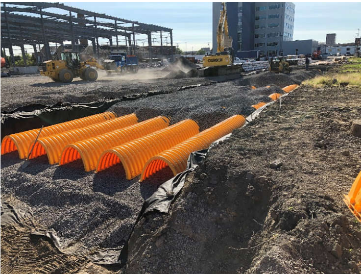
Construction of the underground infiltration system at the Ranalli ALA project
