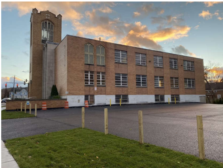
Post-Construction photo of the completed porous parking lot
