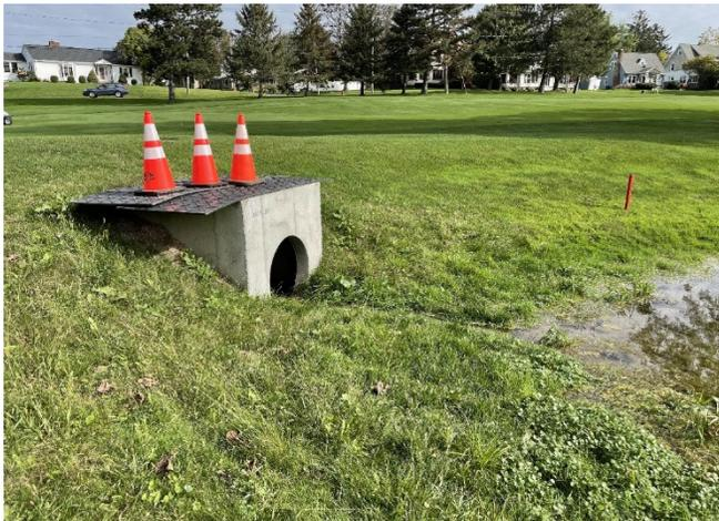
Post-Construction photo of the new overflow structure for the lower pond
