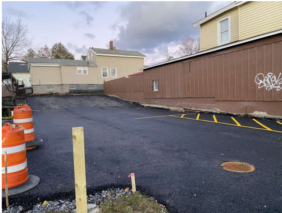
Post-Construction photo showing porous pavement parking lot
