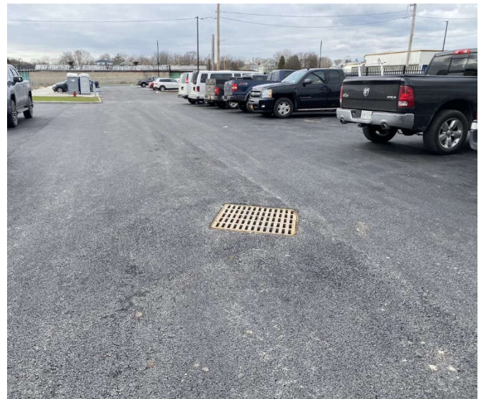
Post-construction photo of parking lot above the chamber system
