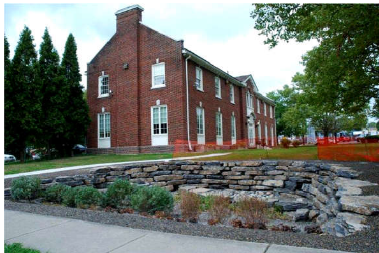
Completed Bioretention Area at White Library
