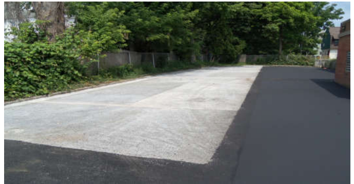
Porous Concrete Area Behind Petit Library
