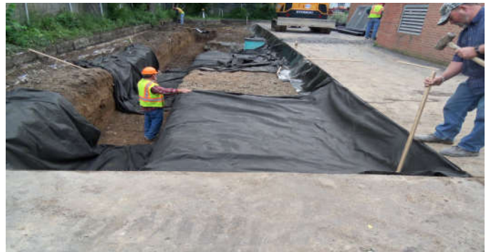
Construction of Infiltration Bed
