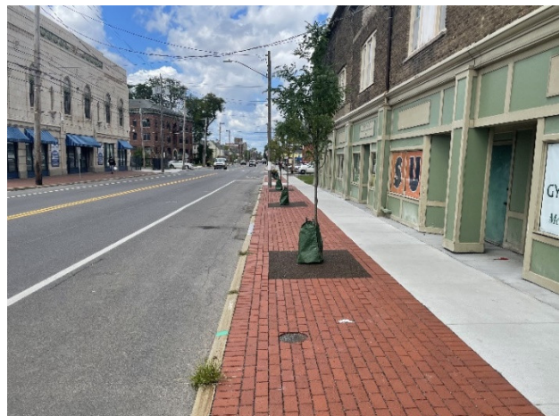
Photo of Completed Tree Trenches; Not Seen are the Subsurface Silva Cells Pictured at Left
