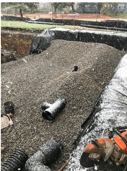
Beneath the Basketball Courts
