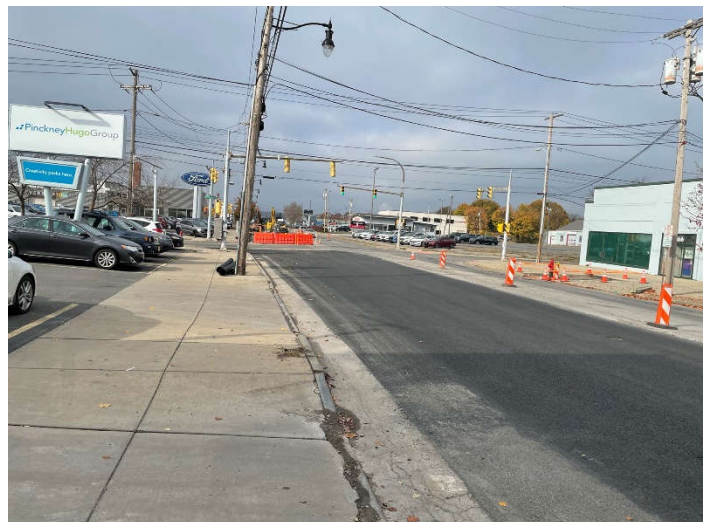
Post-construction infiltration trench location after initial paving
